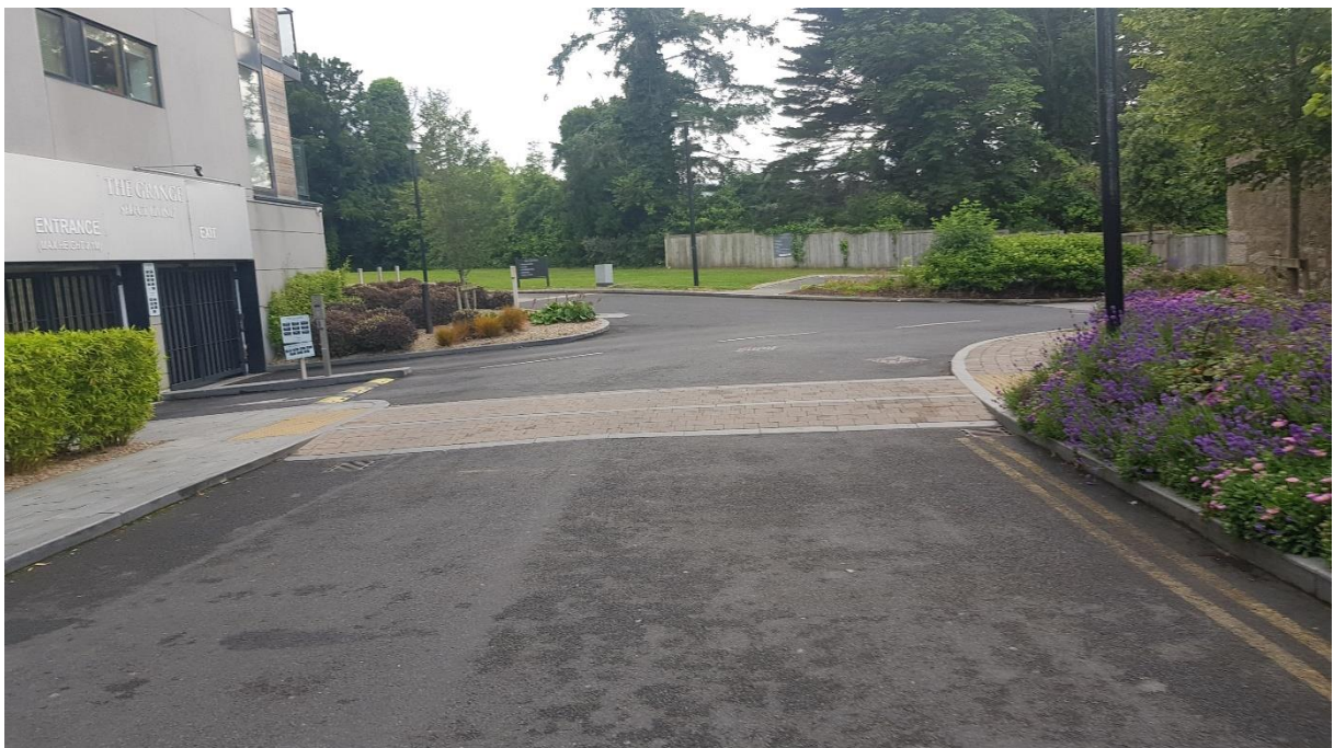
Figure 51: Existing raised crossing & Speed Bump at Car Park Access
