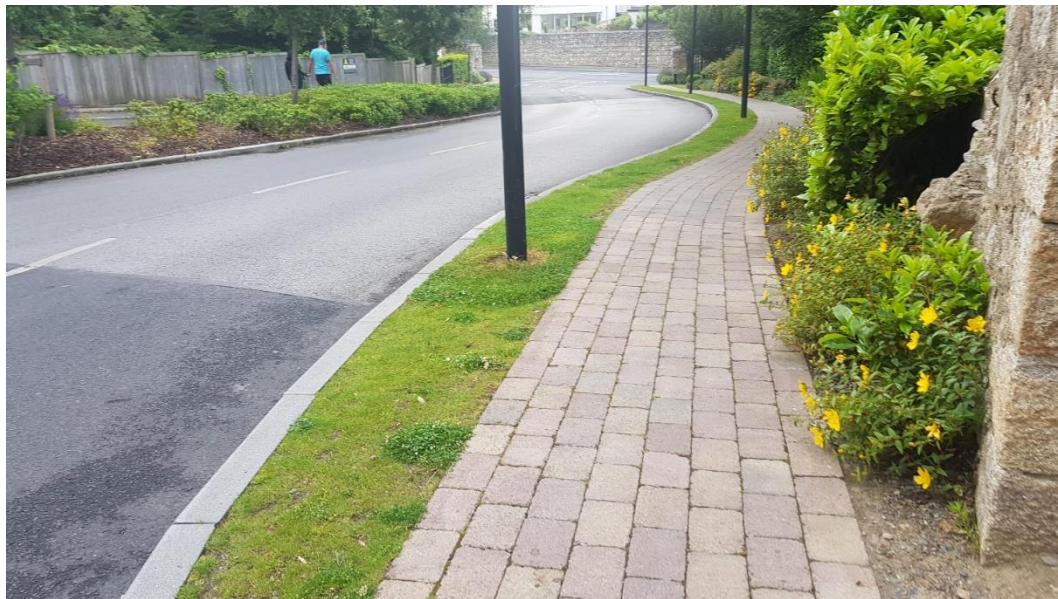
Figure 70: Connectivity to narrow Existing Footways Unclear
