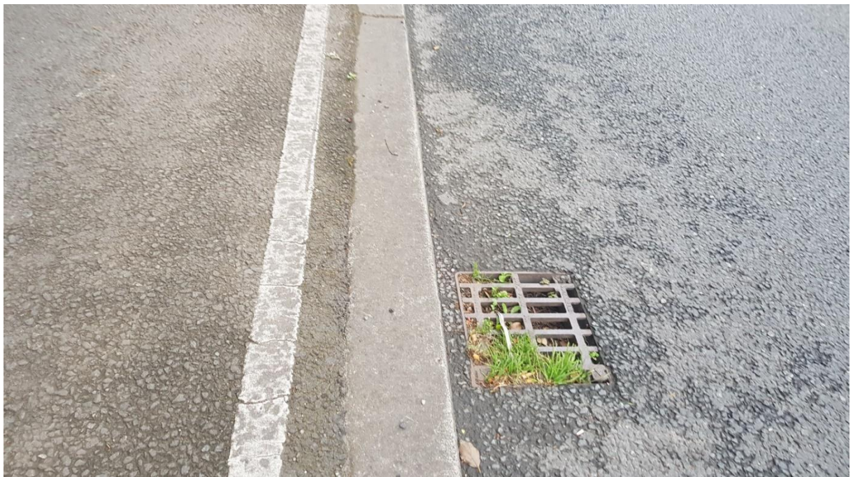
Figure 43: Blocked Gully on N31 adjacent to site
