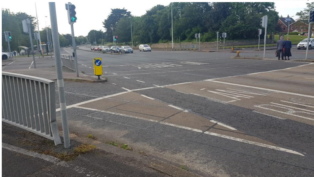
Figure 33: Signs and Guardrails Struck
