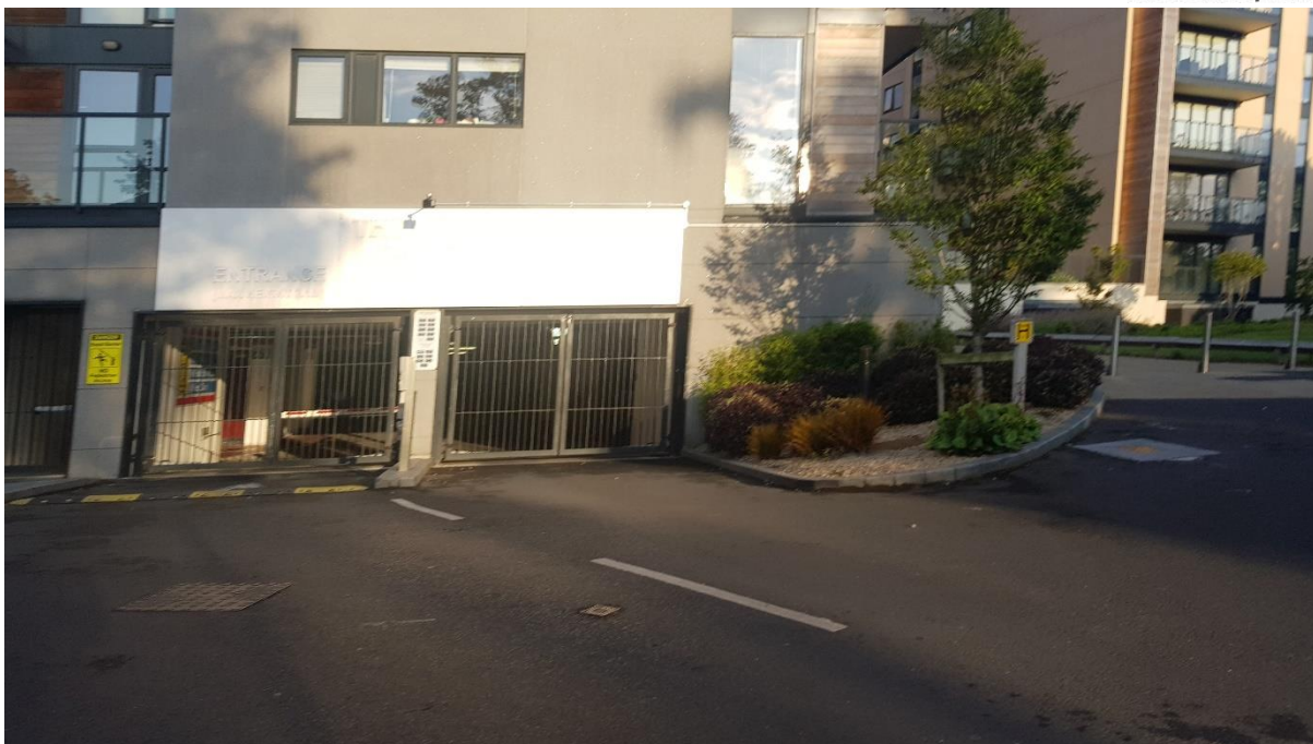
Figure 52: Existing Speed Bump at Car Park Access
