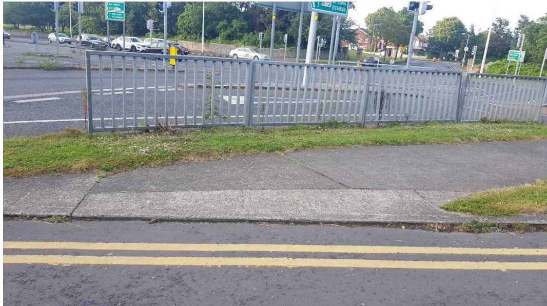
Figure 37: Tactile Paving Absent
